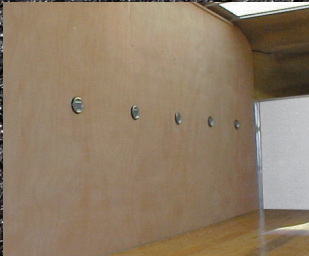
Plywood lining with D-rings
